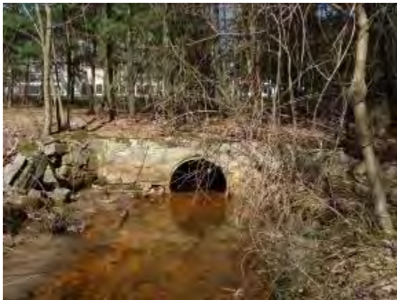
Two views of storm drainage from Evelina Drive and red stream bed (product of iron-loving algae not pollution)
